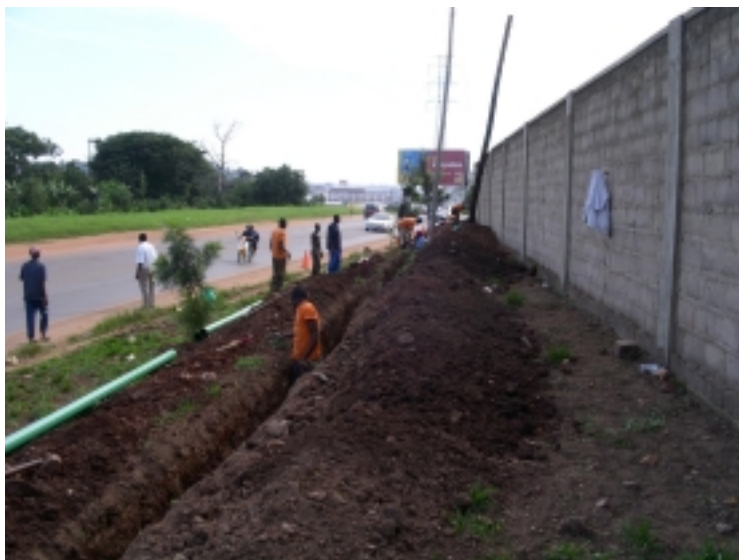
Figure 8: Fibre Optic cable being installed for MTN in Kampala, May 2005
